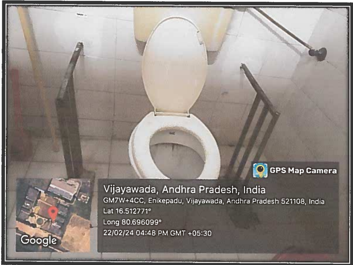
Toilet for Divyangjan
